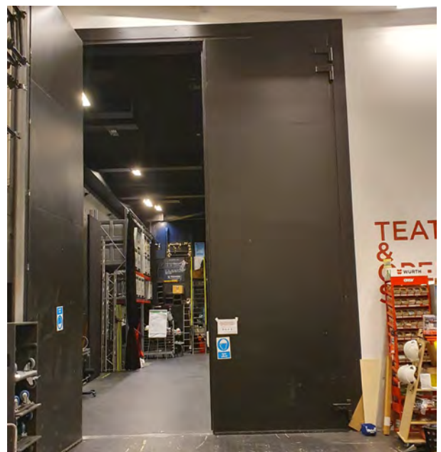
Stage Fire Door
