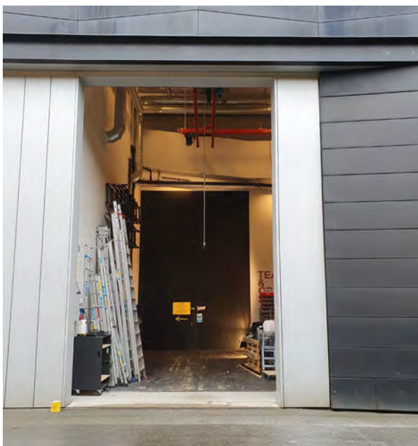
Loading Bay Door
