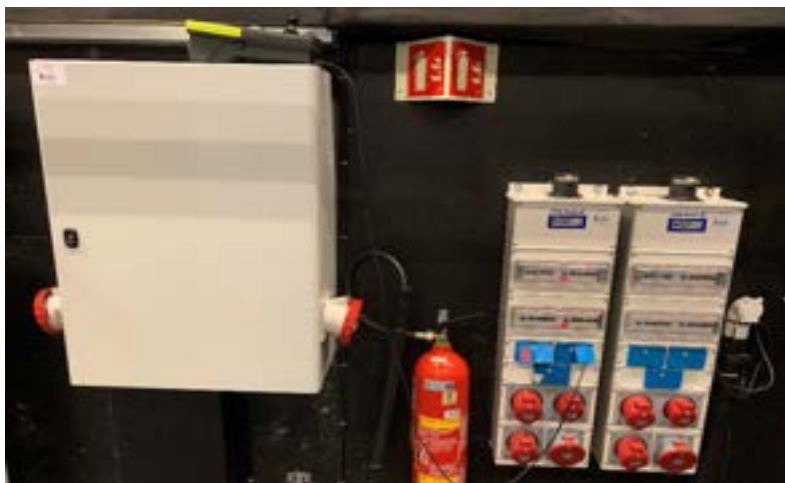
125 A 3 p and 2 x 63-amp boxes stage right.
