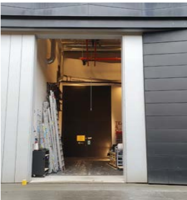
Loading Bay Door
